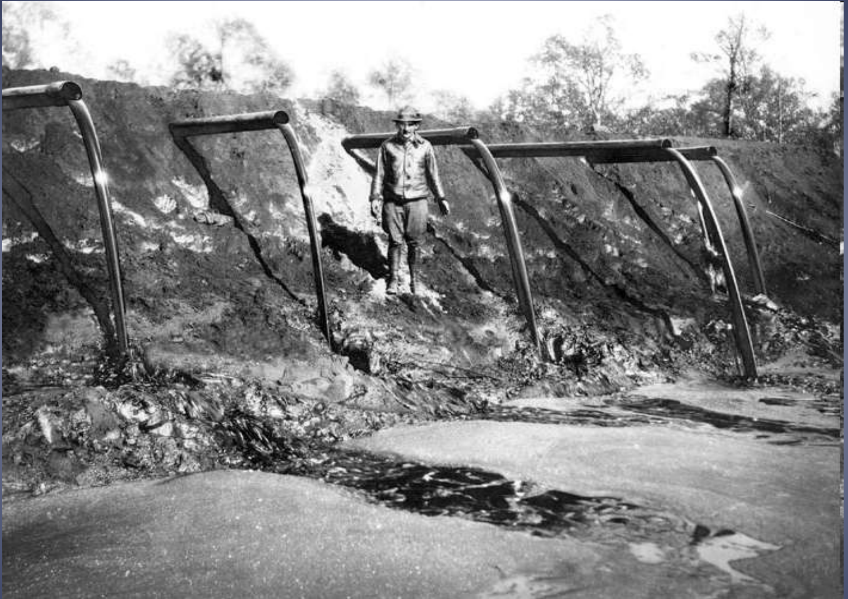
Flow from the Otto Morris and Marr Oil Well Flow, an oil well in south Arkansas. Earthen storage pits were used for the crude oil. From 1922 to 1934, up to eight percent of the oil produced was wasted, and almost all of the natural gas escaped. ( http://encyclopediaofarkansas.net/encyclopedia/entry-detail.aspx?entryID=383# )
