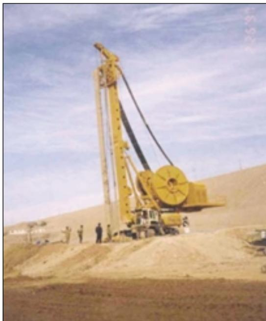
Excavation of the cutoff wall in the riverbed by a BC30 Cutter.
